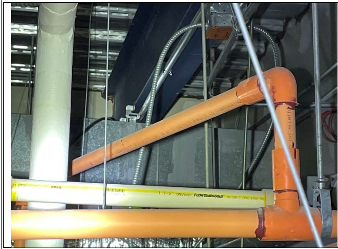
Photo 35: HM-HH: Duct Mastic, Gray
